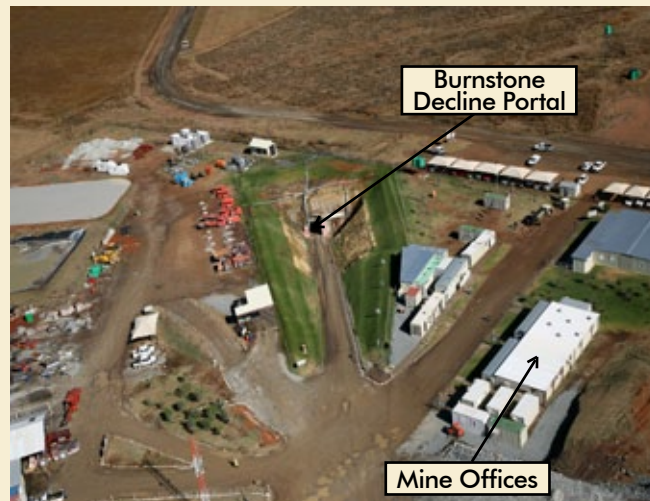
Aerial view of the decline portal at Burnstone mine
